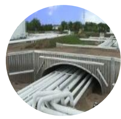
Inside Culvert, underground structure
