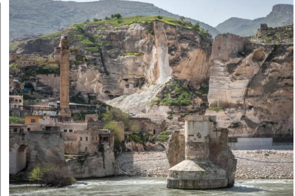
Landslide due to flood
