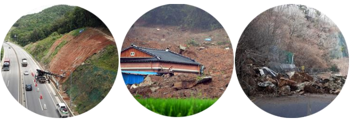
Roadside with steep slope, Landslide, Falling Rocks, Old Embankment & Bridge
